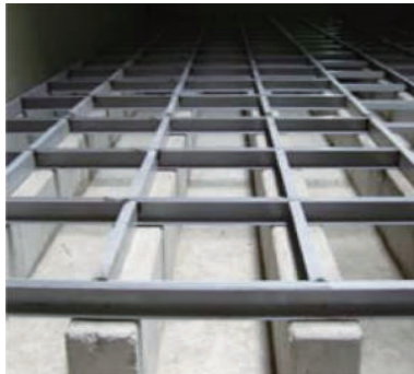
Installation of Base frame pad
