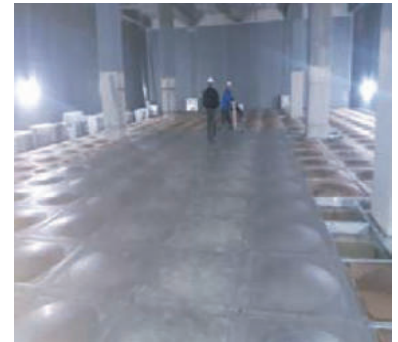
Installation of bottom plate
