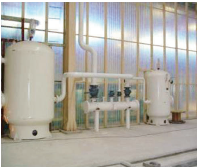
AIR RECEIVER TANK
