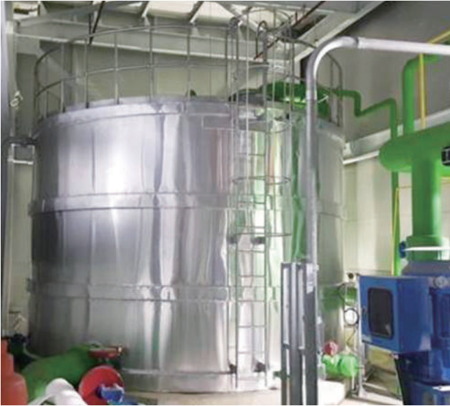
CONDENSATE WATER TANK
