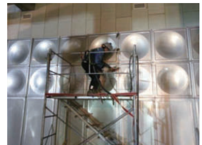
Side plate installation
