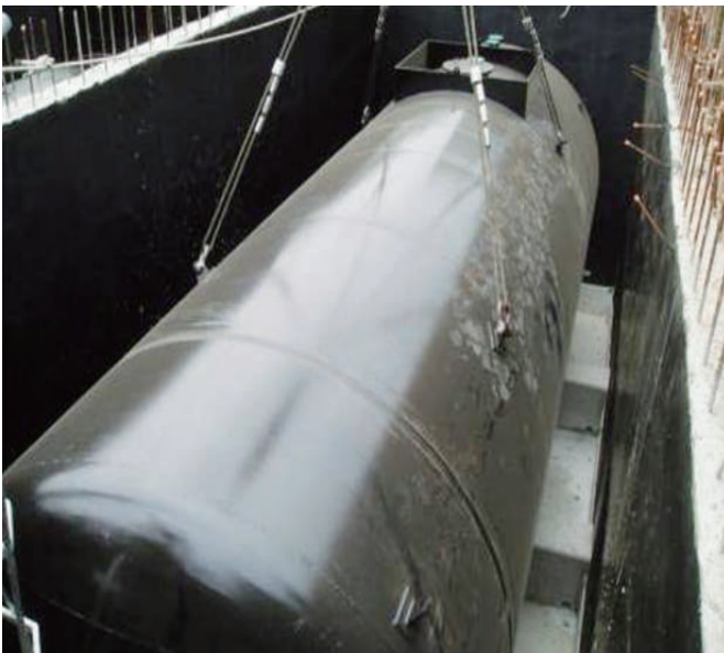
BASEMENT STORAGE TANK
