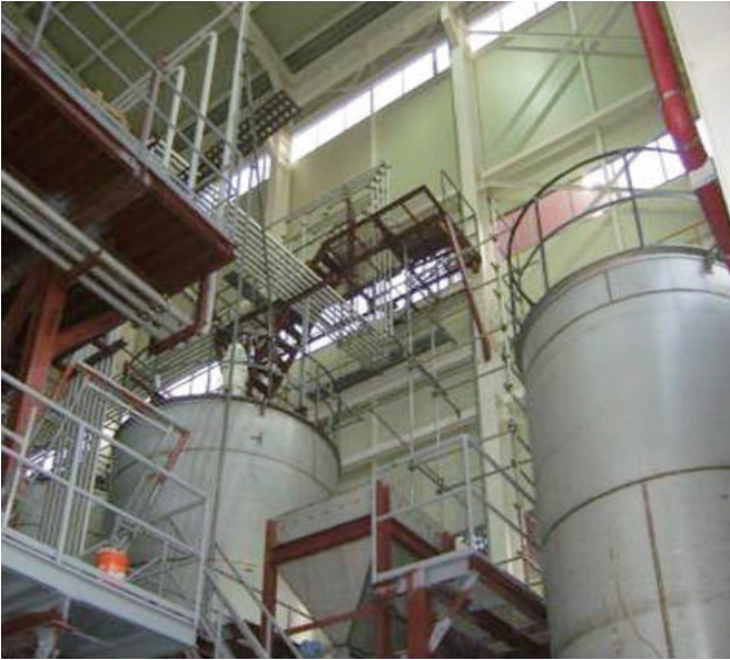
BIOCIDE STORAGE TANK
