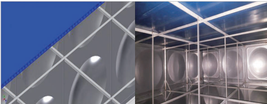
Intersecting angles to prevent sagging
