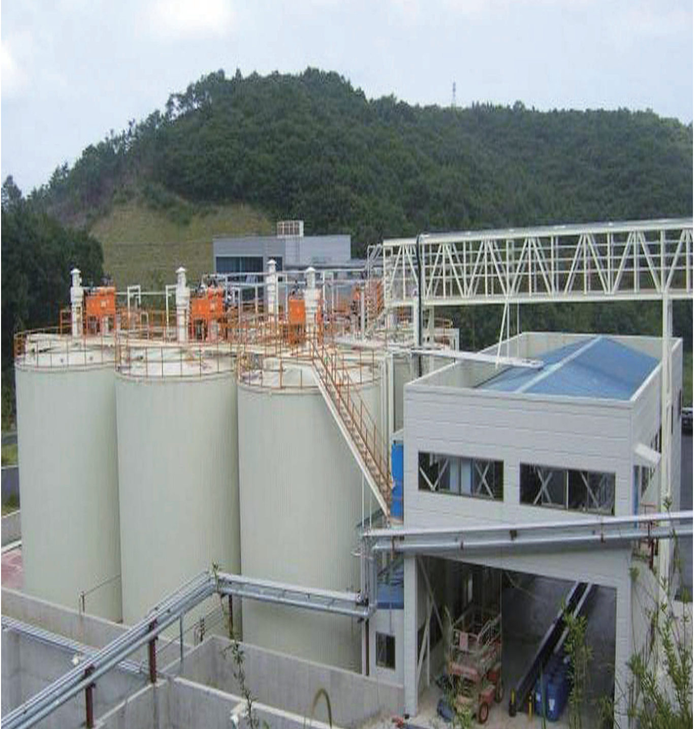
HEAVY CALCIUM CARBONATE TANK & PIPING LINE 50 UNITS INCLUDING 500 TON
